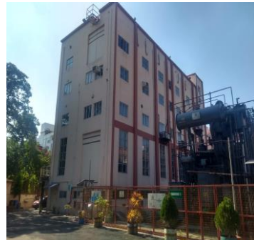
B T Road SS – Certified LEED v 4.1 Gold in 2023 by USGBC
