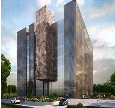
RPSG House – Certified as “LEED (v 4.1) Platinum in 2023 by USGBC
