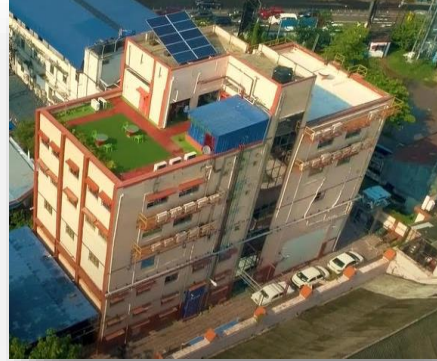
Park Circus Substation – Certified LEED v 4.1 Platinum in 2022 by USGBC
