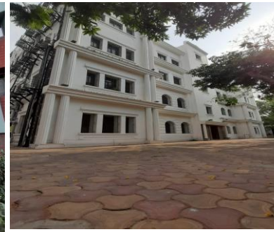
Lord Sinha Road Office – Certified as LEED v4.1 GOLD in 2023 by USGBC
