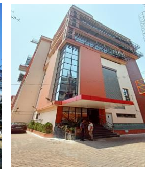
Lord Sinha Road Office – Certified as LEED v4.1 GOLD in 2023 by USGBC
